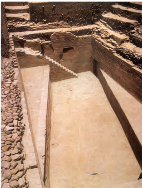
Fig. 1.5 Reservoir at Dholavira Note the masonry work.
